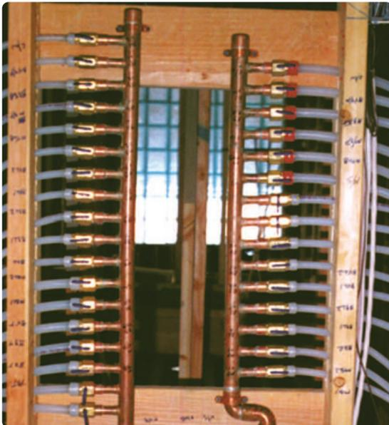
Uponor ProPEX Valved Manifolds run individual hot and cold water lines to each fixture, reducing pressure and temperature swings.
