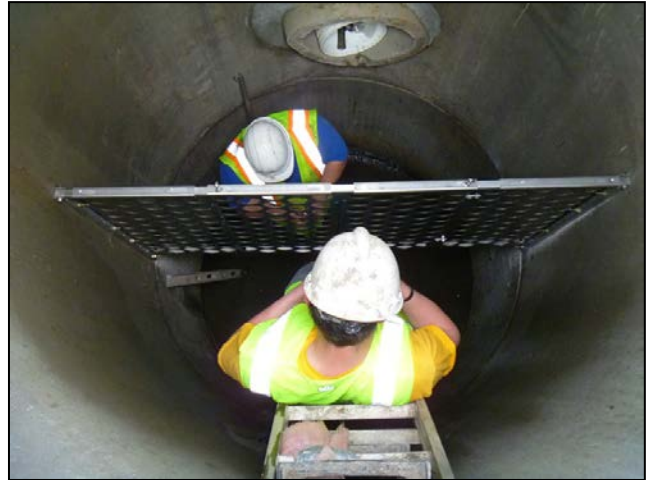
The SAFL Baffle, developed out of the University of Minnesota College of Science and Engineering’s St. Anthony Falls Laboratory (SAFL), keeps sediment pollution out of lakes, rivers and oceans.
