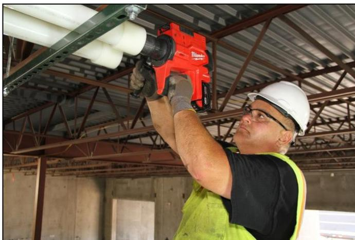
Uponor's new offering of PEX pipe and ProPEX® expansion fittings in 2½" and 3" sizes includes Uponor AquaPEX® pipe for potable-plumbing applications and Wirsbo hePEX™ pipe for hydronic heating and cooling applications.
